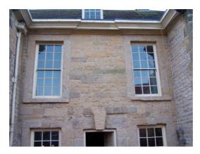
A similarly architraved stone window was added to the west wall, probably occupying an already altered opening that originally contained a medieval solar window. A new stone doorway was added from the central range to the garden, this time within the arch and at right angles to it, in the west wall of the 'H'. A new stone window with semi-circular head, reflecting that of the arch, was added to the stairs in a newly made, or what may by that time have been an already existing, opening.
