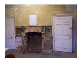
Major reconstruction work took place at the west end of the building, associated primarily with the introduction of flues, and especially of the massive flue of the kitchen fireplace. The huge 3-centred arched Hildenley limestone fire surround that this flue served was probably introduced at this time and may well have been pilfered from the Priory kitchen.
