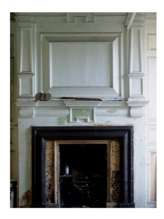
The wainscot covered earlier decorative finishes: earth plaster beneath a haired lime finish coat and limewash, which remains today. The central great chamber over the hall was fully wainscoted and continued to be entered at the head of the stair.
