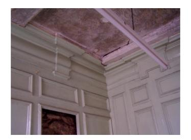
The south panelled wall was moved to its current location in the mid C18, mounted on a stud wall of this period, creating a separate landing from which the cross wings are now accessed and disrupting the effect of the earlier (and probably original) 9-bay coffered ceiling
