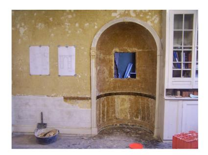
It is formed of lath and plaster and retains (beneath modern lining paper) all coats of paint applied to the walls of this room, but since removed everywhere else. It is unlikely that this removal could have been carried out to the C18 plaster without seriously damaging it, and this has not occurred. It pre-dates the plaster. A similar colour sequence survives upon the unusual low level panelling, which is formed of long horizontal boards.
